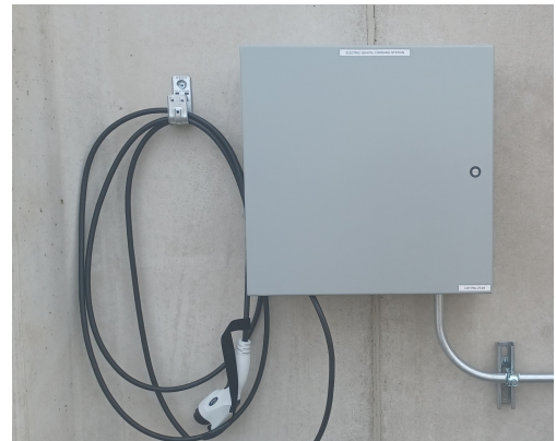
(c) Level 2 AC 220-volt charging station
